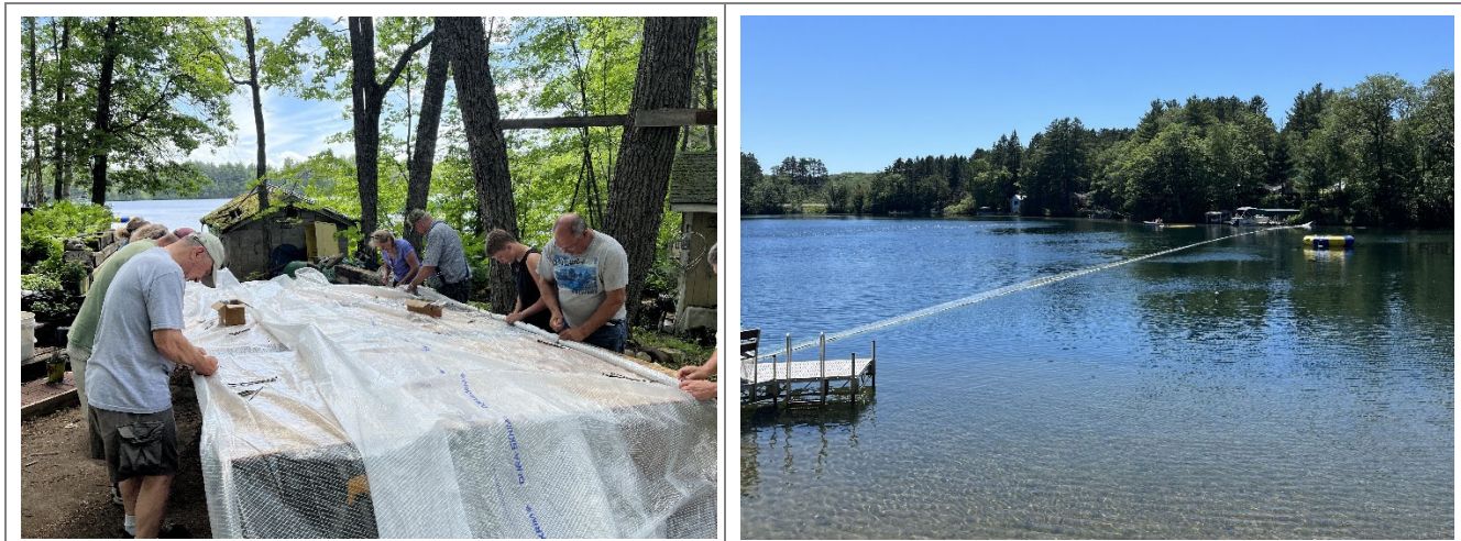
Photograph 3.1-1. Barrier curtain construction & placement in Twin Bear Lake. Photo credits IRPCLA.
